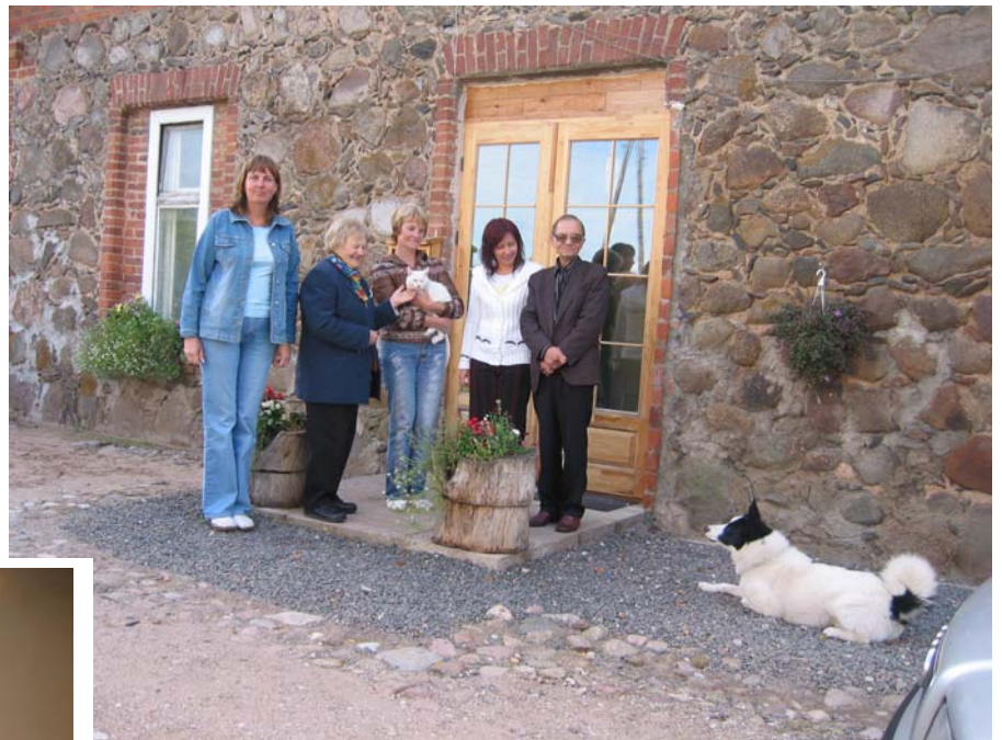
The congregation at Umurga is currently restoring the parish manse. (the front door of the manse – with visitors!)
